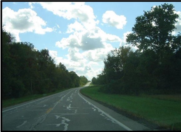
State Route 61, a mid-county north-south corridor
