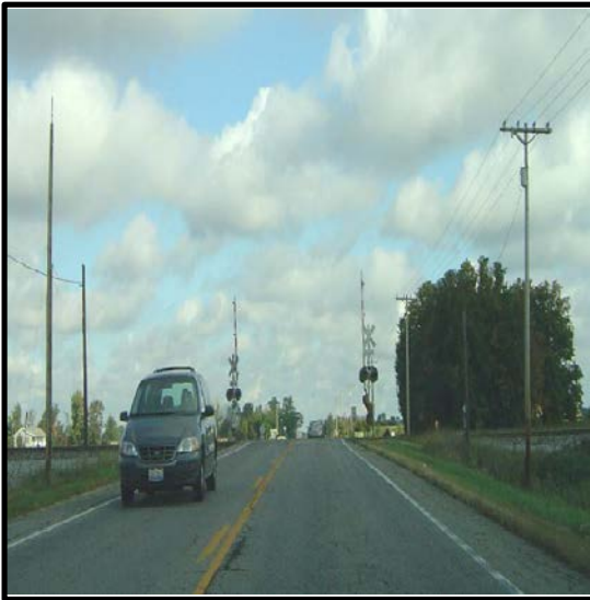
Grade crossing along SR 13 near Greenwich, slated for a Grade separation improvement.
