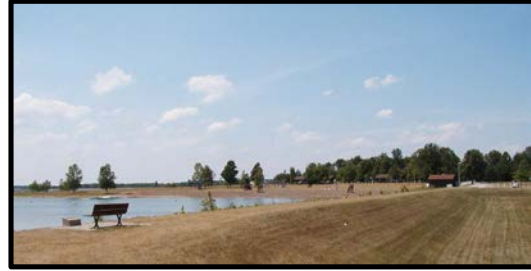
Scene at the New London Reservoir
